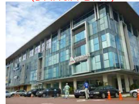
施工場所② ISKANDAR REGIONAL DEVELOPMENT AUTHORITY (DANGA BAY)
